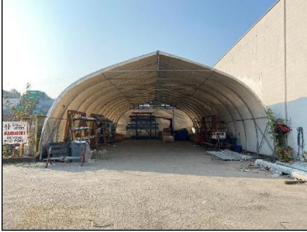
Photo 5 Anthropogenic structures on the property. No evidence of nesting birds was observed. (2022-10-18)
