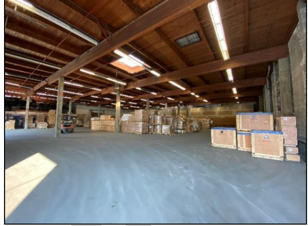
Photo 6 Interior of main warehouse on the property. No evidence of nesting birds was observed. (2022-10-18)
